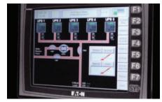
The touch-sensitive SBM display shows a graphical view of a large parallel system with intuitive controls and quick access to key information like battery time remaining and event/alarm history.
